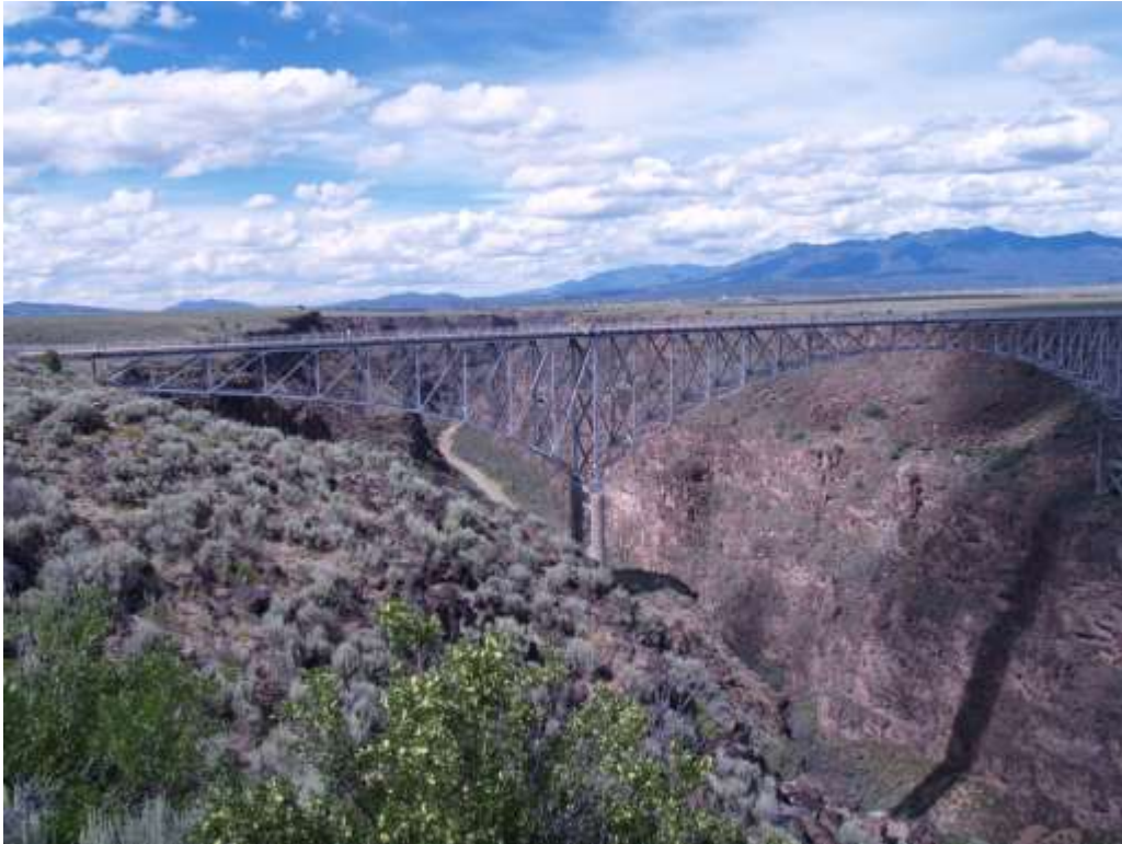
RIO GRANDE GORGE BRIDGE, NEW MEXICO
